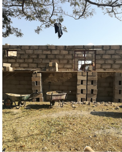
Figure 4. One wall of the house volunteers helped to build.
